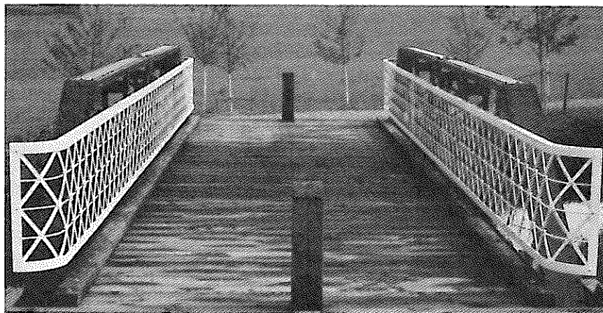
FIGURE 5 A low Warren truss bridge removed from a town highway in Hinsberg, Vermont, restored and adaptively reused as a pedestrian bridge at another location in Hinsberg. (Vermont Agency of Transportation photo)
